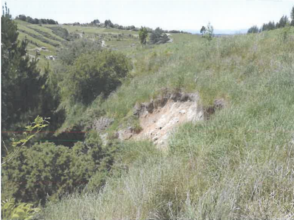
3.1 Slump 1 north of ROW P; Lots 9/10 (view looking east)
