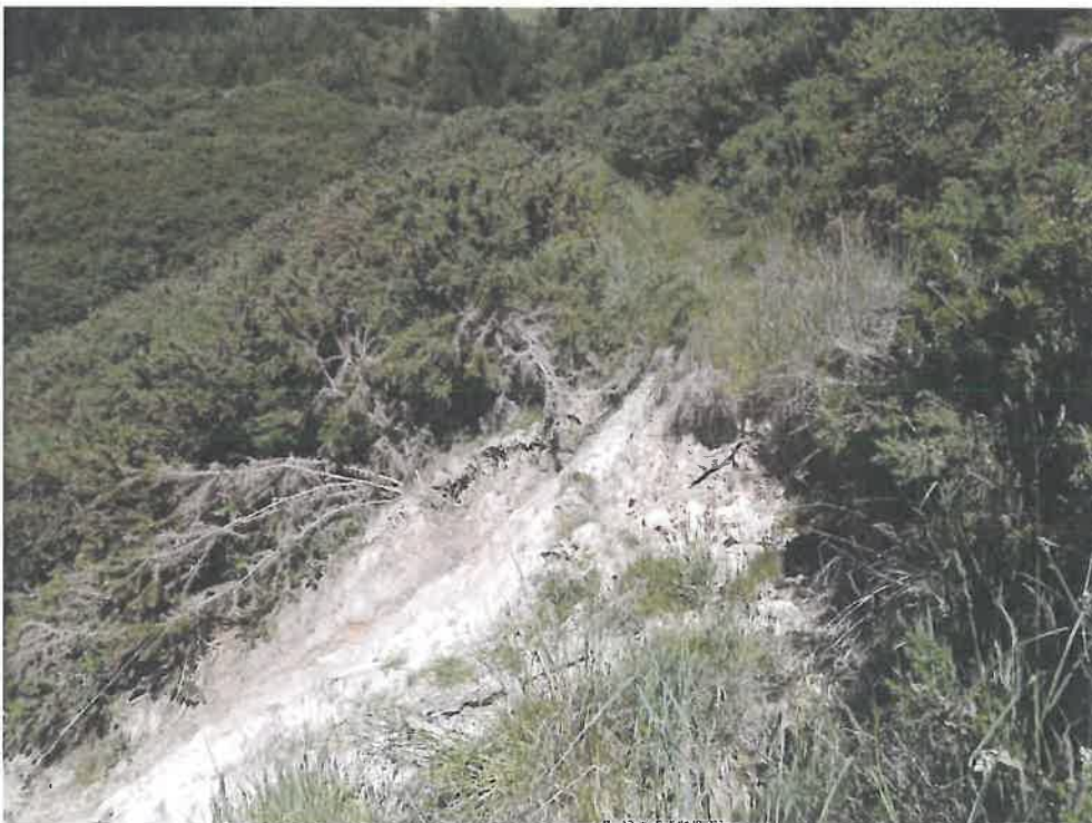
3.2 Slump 2 east of ROW C; Lots 10/11 (view looking south)
