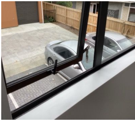
The window stay in bedroom two needs re-attaching.
