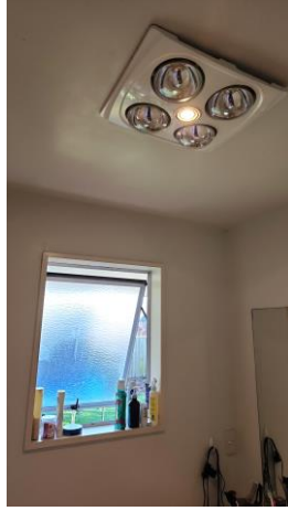
Bathroom 2 Install spacer soon.
