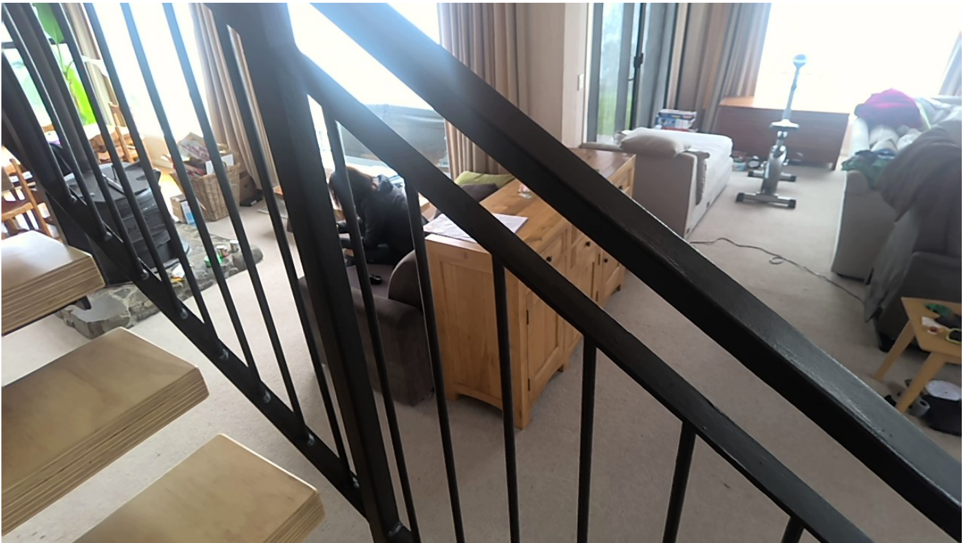
Handrail and barrier
