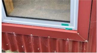
This may be to stop wind driven rain entering. Caps can be sought and fitted to stop this problem. There is minor staining to the reveals of these windows.
