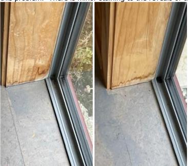
There appeared to be no current leaking and no elevated moisture levels (using a non-invasive moisture metre) to the interior.
