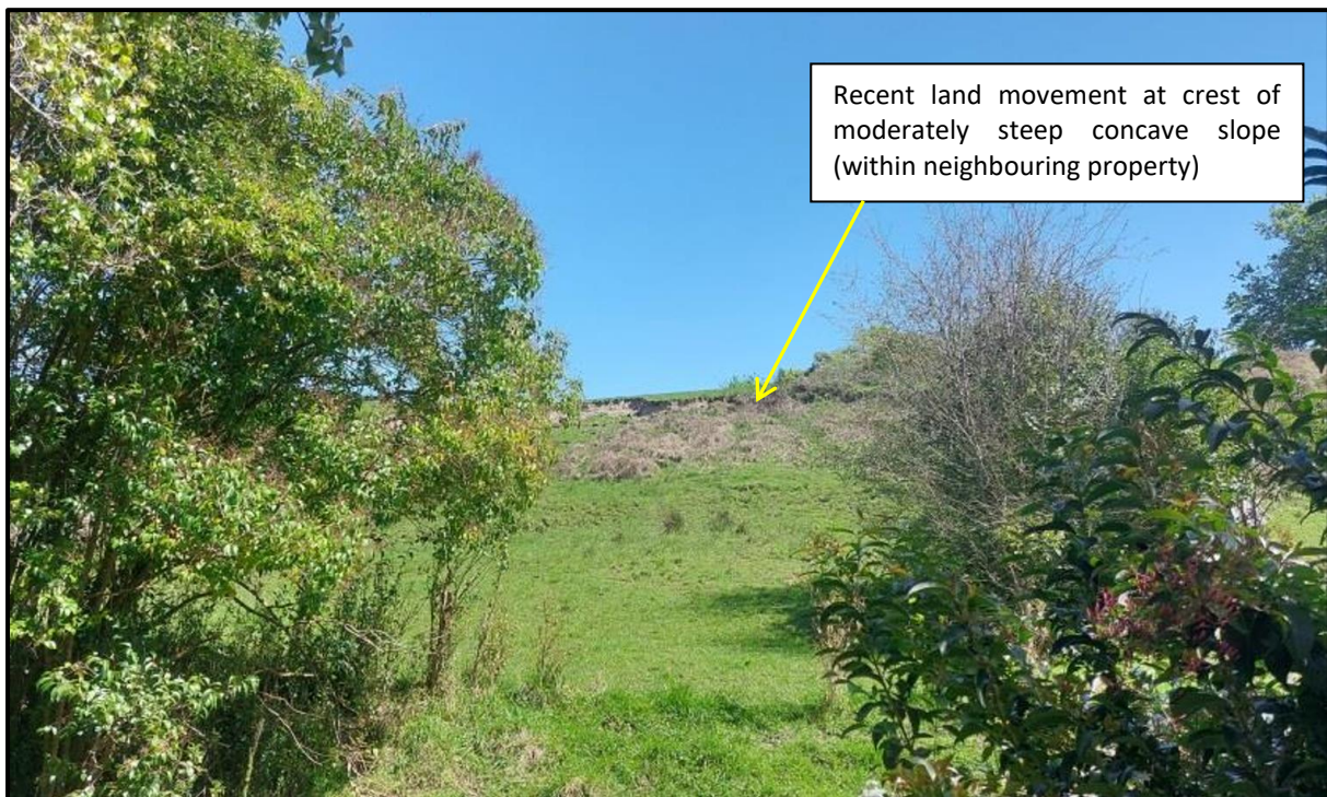
Figure 2: Land Movement at Crest of Concave Slope in Neighbouring Property
