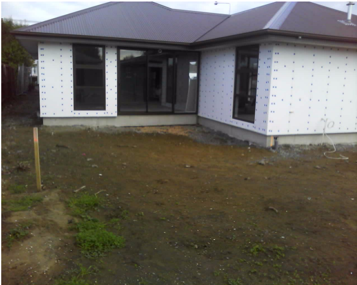
WANZ bar still to be installed to sectional slider Taken at 10:09 AM on Tuesday 19/05/2015
