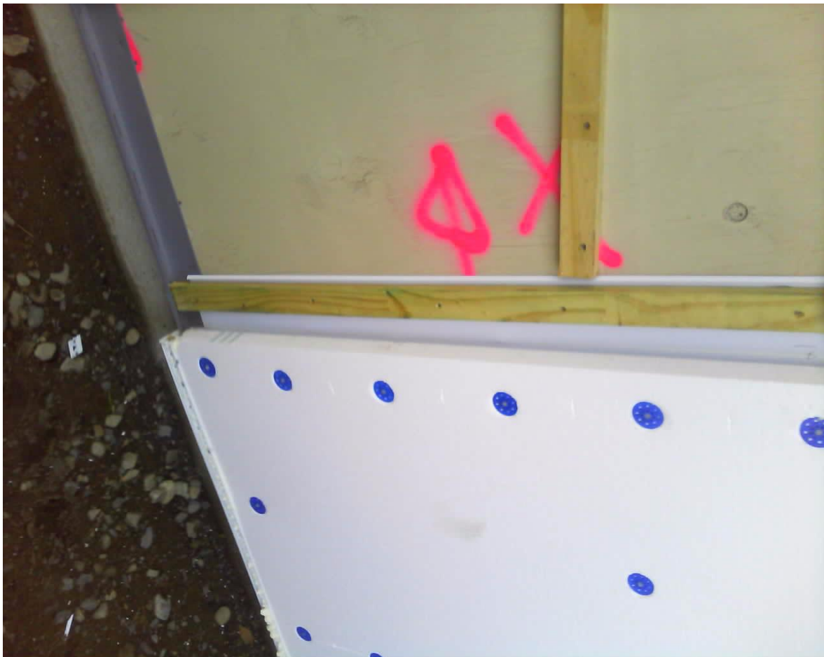
Change of cladding back flashings Taken at 10:00 AM on Tuesday 19/05/2015
