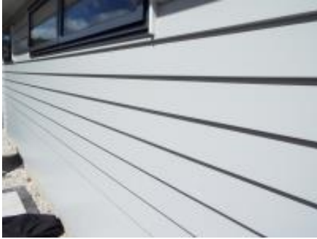
exterior well painted
