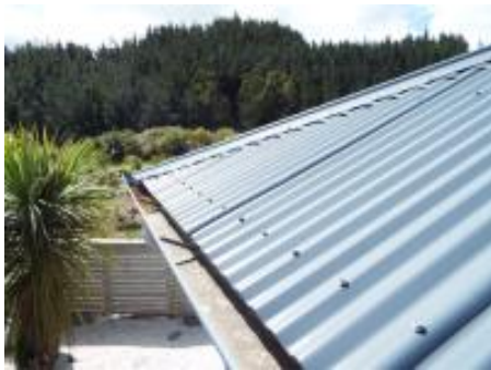
gutters clean at the time of inspection
