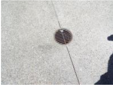
good drainage noted
