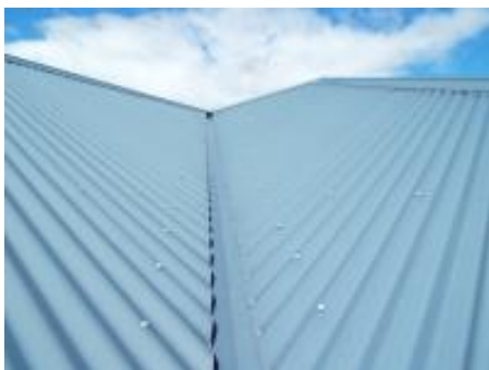
valley flashing in good order
