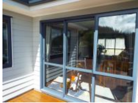
joinery in good working order
