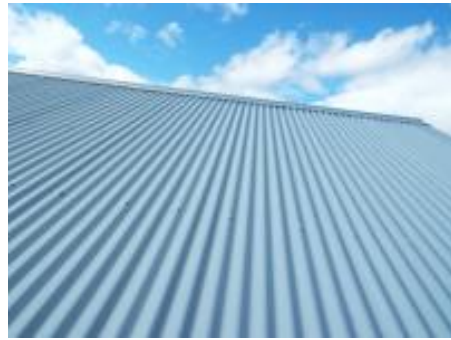
roof clean at the time of inspection
