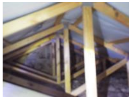
all dry at the time of inspection
