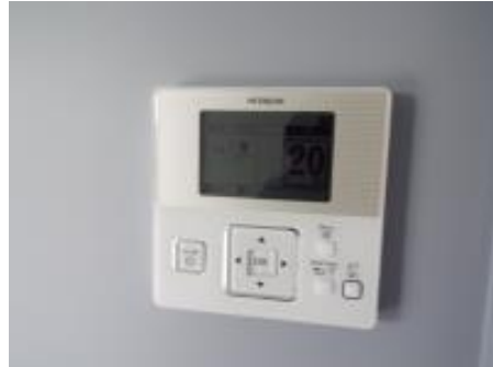
working at the time of inspection
