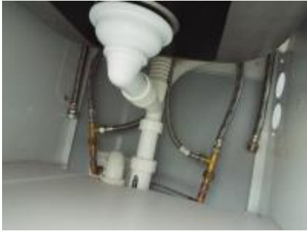
plumbing all good at the time of inspection
