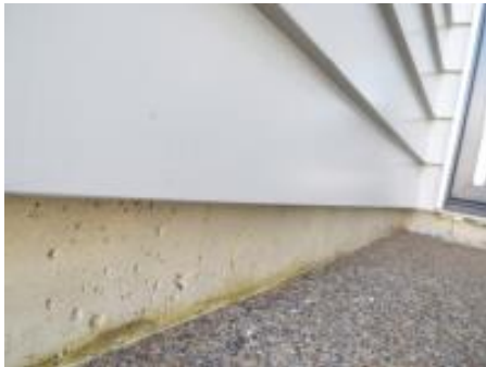
concrete slab in good order
