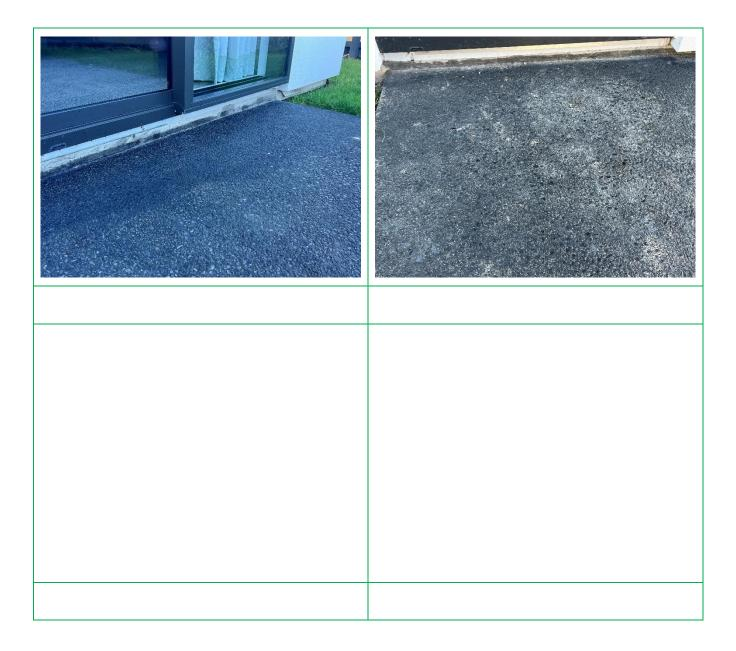
**Recommendations:** Ground and garden levels should be kept below and clear of the cladding and finished floor heights to minimise water ingress, unless specialised drainage is installed the current standards taken off the floor are A min of 150mm to permanent paving and 225mm to unprotected ground
