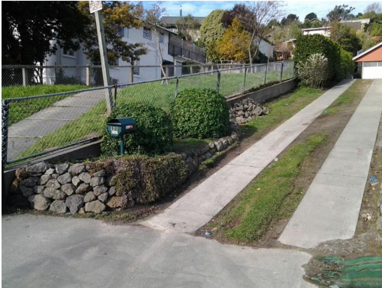
Elevation of wall 5 on the LHS boundary from the road
