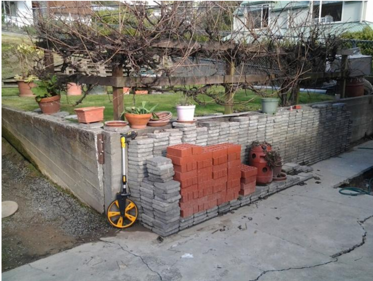
Elevation of wall 6 behind the house
