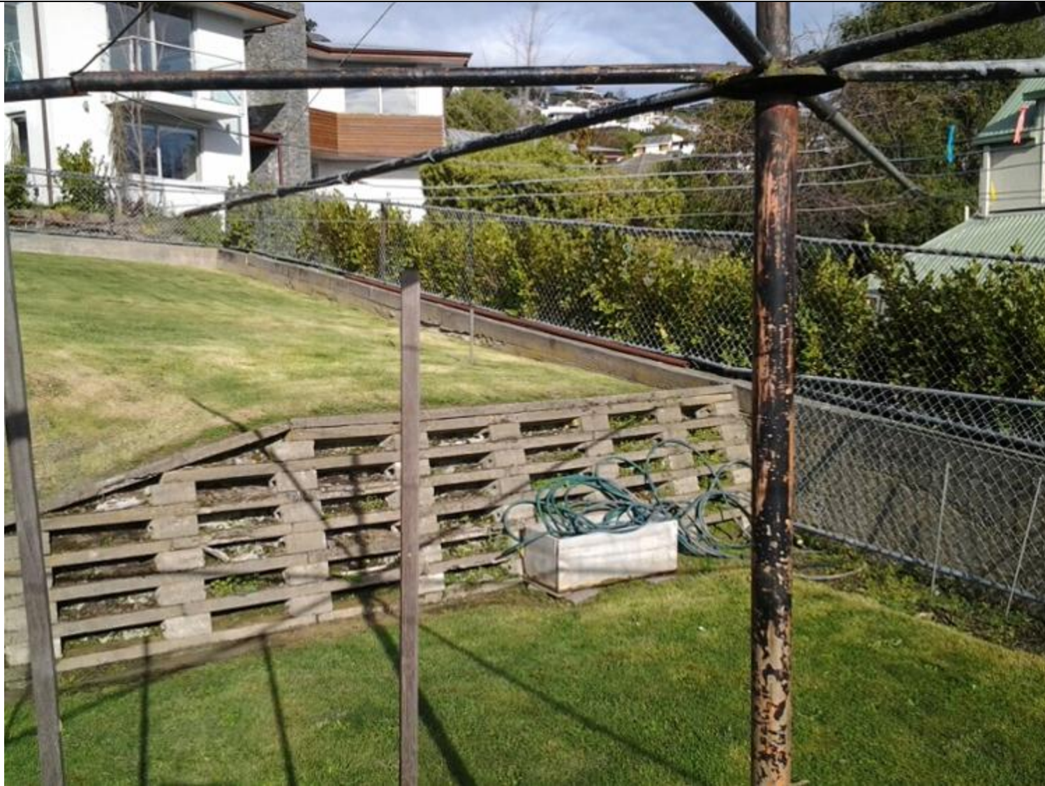
Elevation of RHS of wall 5 from the upper garage
