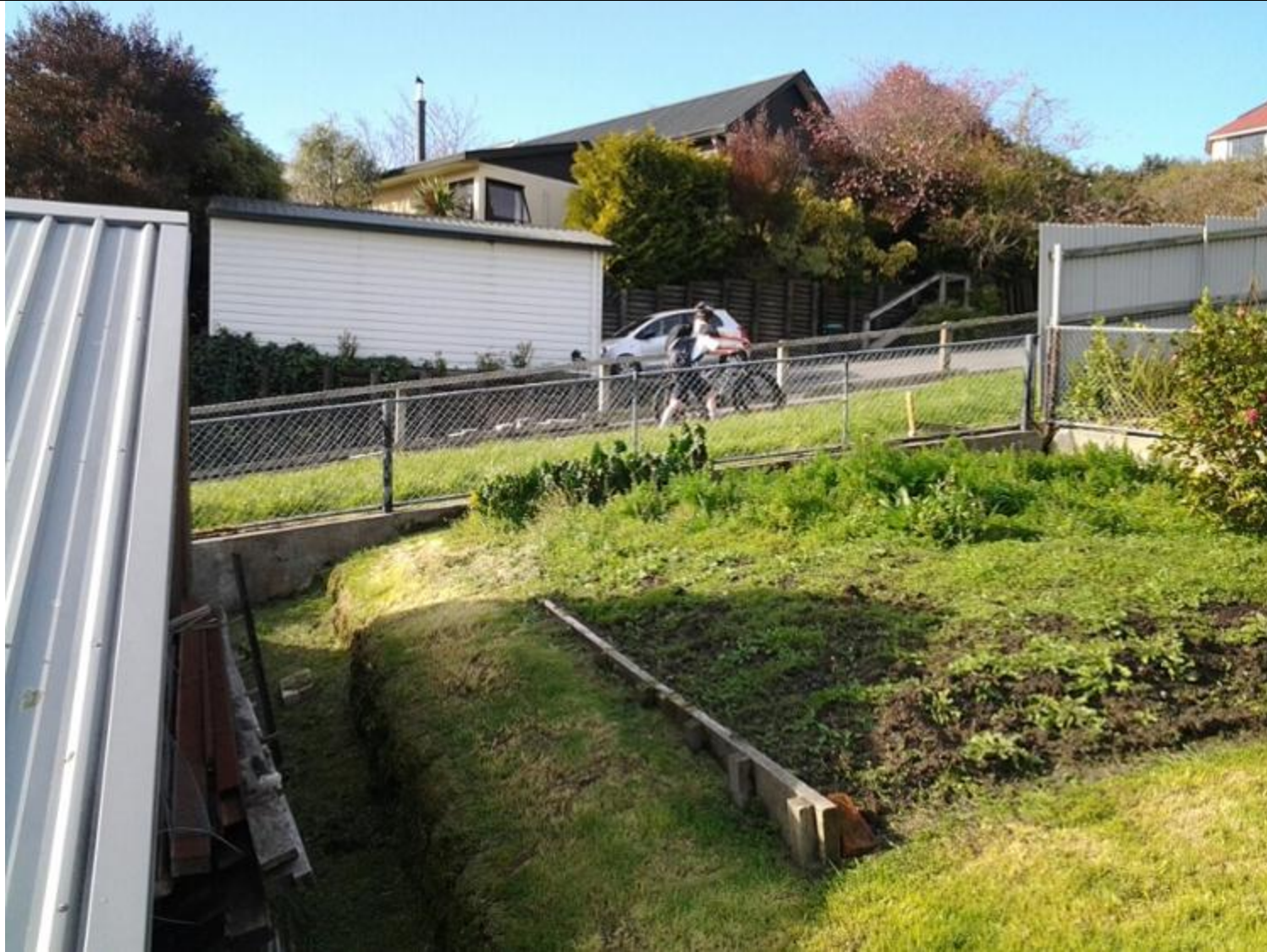
Elevation of wall 5 on the LHS behind the upper garage
