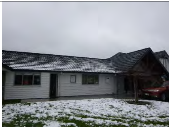
Photo 1: Managers' residence south elevation
