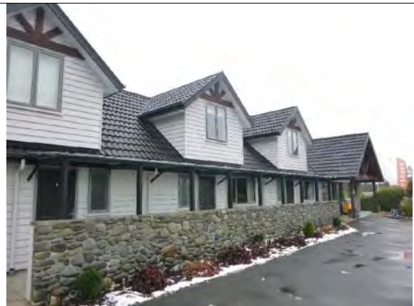
Photo 2: Adjoined apartment wing south elevation
