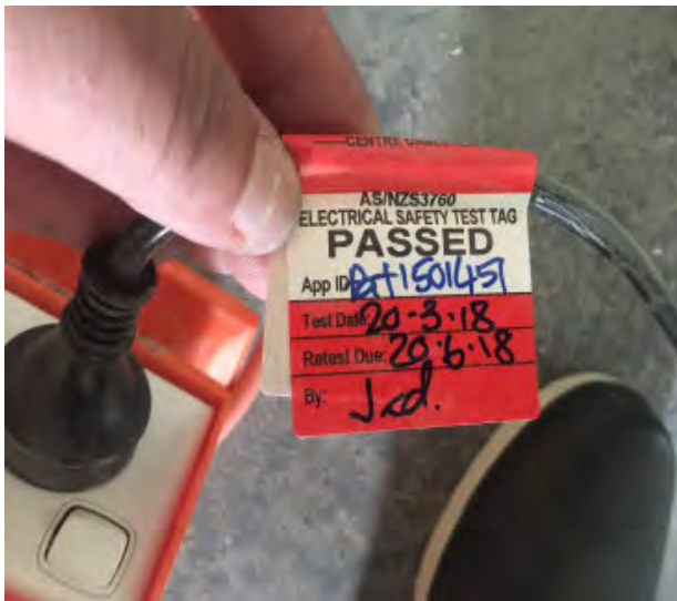
Up to date electrical test tag
