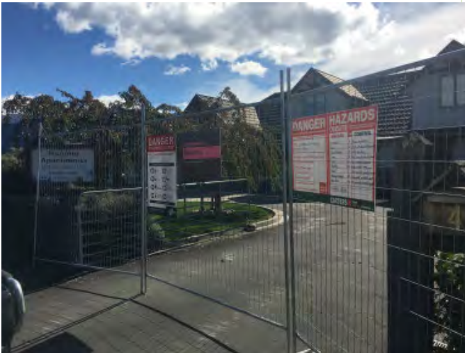
Site fencing/signage erected
