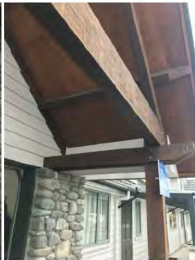
10. South elevation soffit above garage
