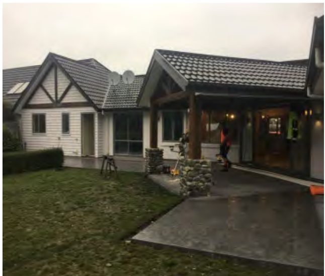
Clean and tidy worksite. Worker in correct PPE
