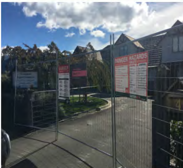
Site fencing, gate, signage
