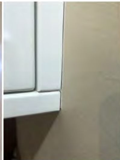
13. Kitchen (1.02) movement to joinery
