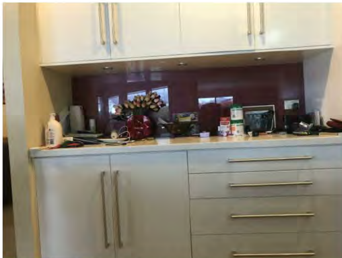
11. Kitchen (1.02) movement to joinery and splash back
