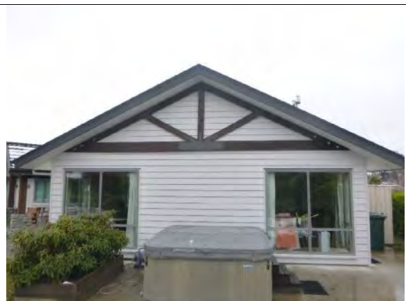
Photo 4: Managers' residence north elevation
