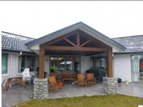
Photo 5: Managers' residence northeast elevation
