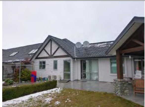
Photo 6: Managers' residence north elevation
