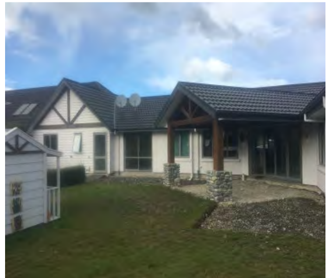
Clean and tidy worksite
