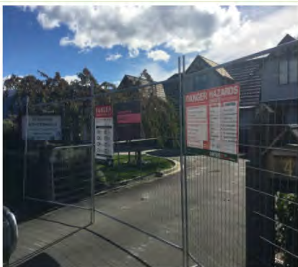
Site fencing, gate, signage, up to date Hazard Board
