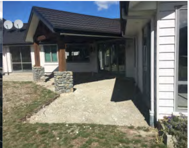
Northern Elevation - Concrete patios and pathways removed
