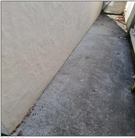
GVB - Subfloor perimeter
