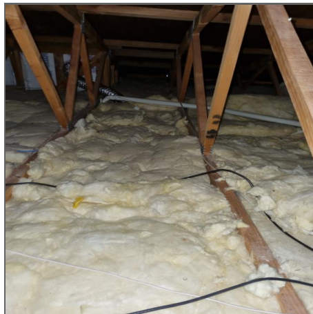
Ceiling - Existing insulation
