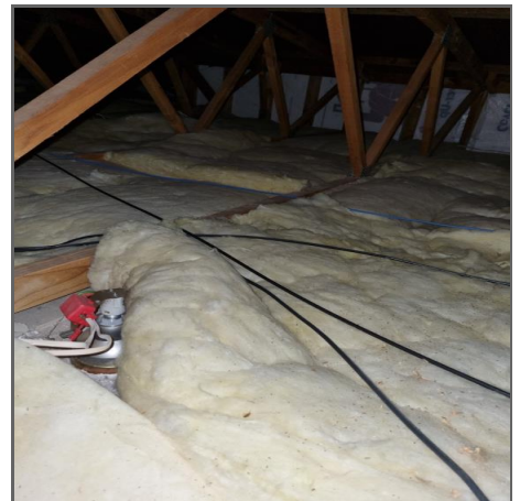
Ceiling - Existing insulation
