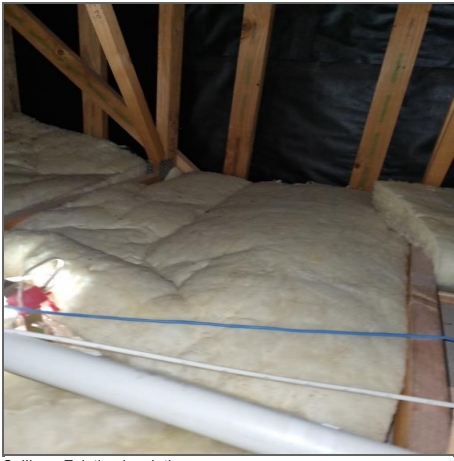
Ceiling - Existing insulation
