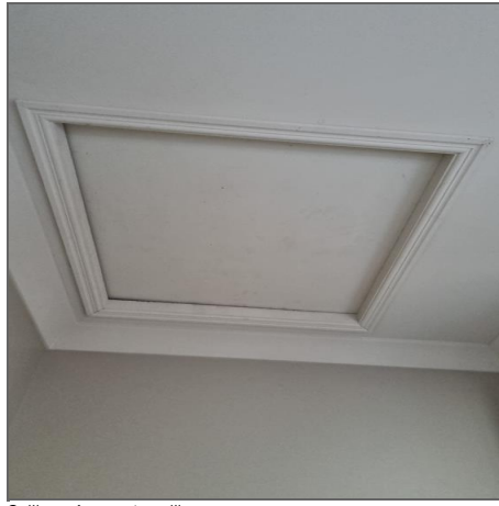
Ceiling - Access to ceiling
