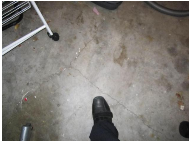
Crack near rear window, ground floor
