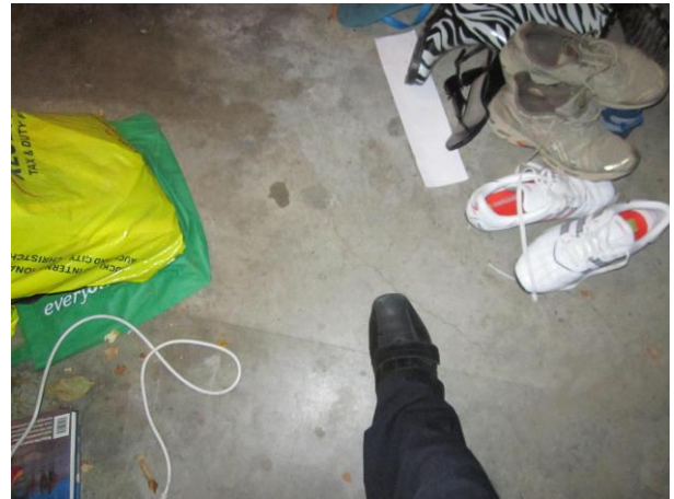
Crack in garage slab
