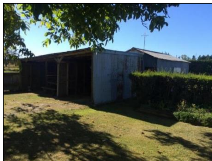
Figure 5: View of the storage sheds at the rear of the dwelling
